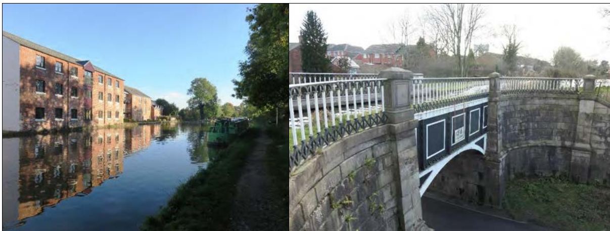
Apartments at the Wharf at the top of Canal Road
