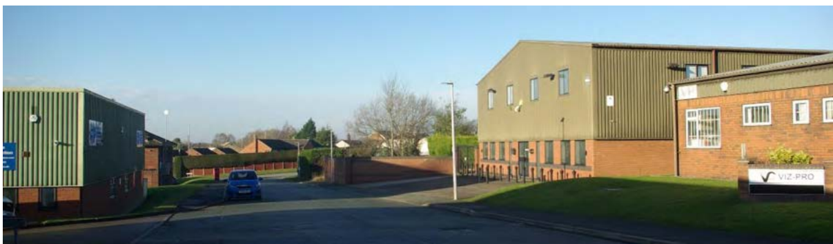
Greenfield Farm Industrial Estate - buildings with recessive green cladding which integrate well into the landscape.
