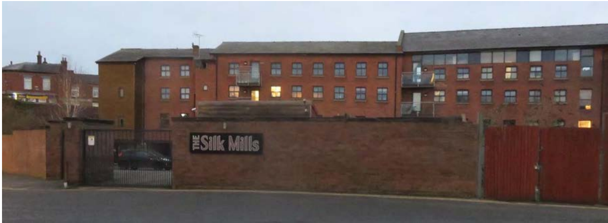
View of Stonehouse Green Mill, one of the 5 former Brook Mills beside the Howty Brook, now converted to housing. The Howty, and associated greenspace, is on the other side of the mill.
