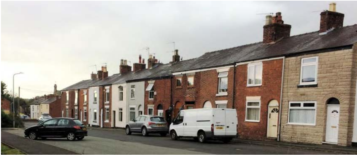
Early C19th terrace on Parson Street near West Road, shown on the Tithe Map of 1838 as part of a large well-established area of densely built streets on a grid-iron pattern.
