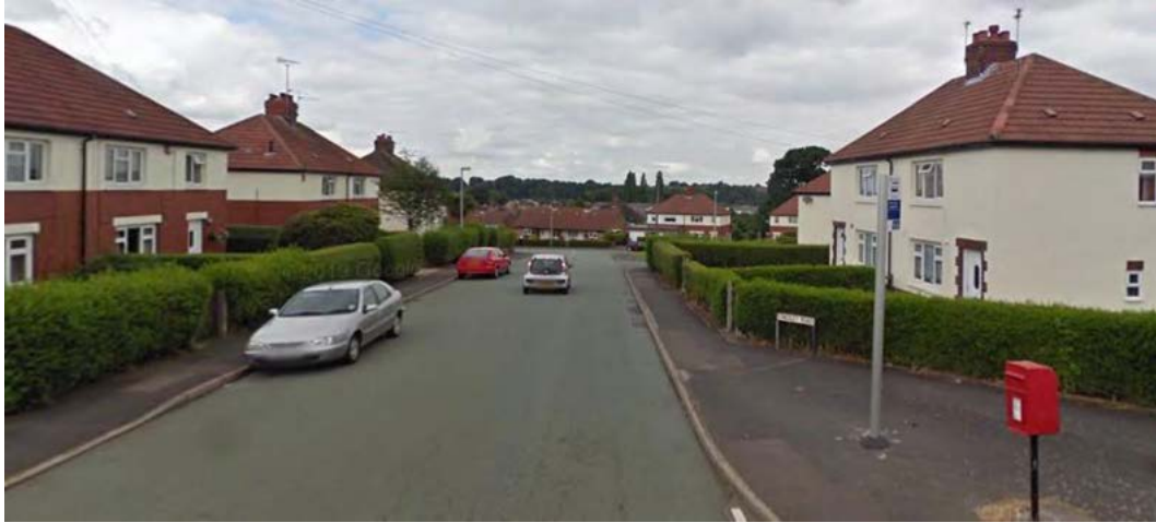
Mid C20th semi-detached planned housing on the Bromley Farm estate, still with privet hedges.
