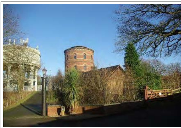
Water towers at West Heath
