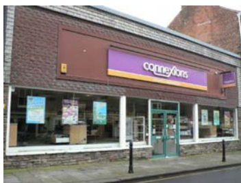
Intrusive 1980s Building used by Cheshire County Council
