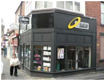
Intrusive Shop Front
