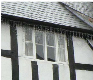
Side-opening Casement in Timber-framed Building
