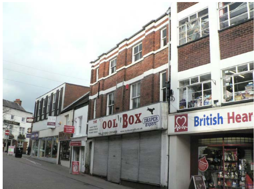
1930s Building at Number 1 Duke Street
