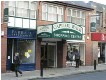
Intrusive Entrance to Capitol Walk Shopping Centre
