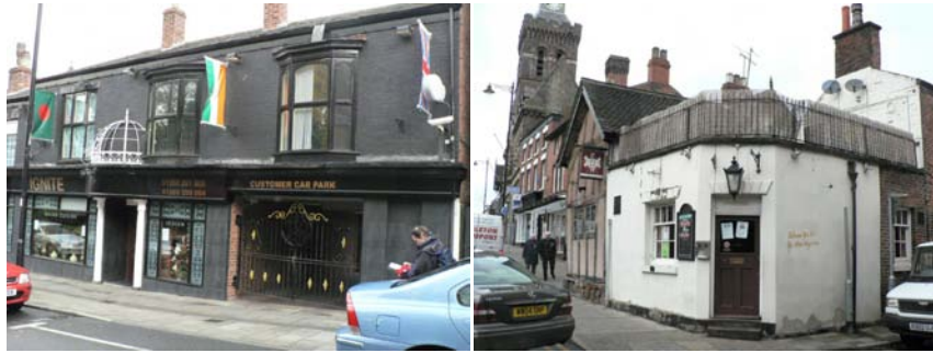
Inappropriate Painted Exterior
