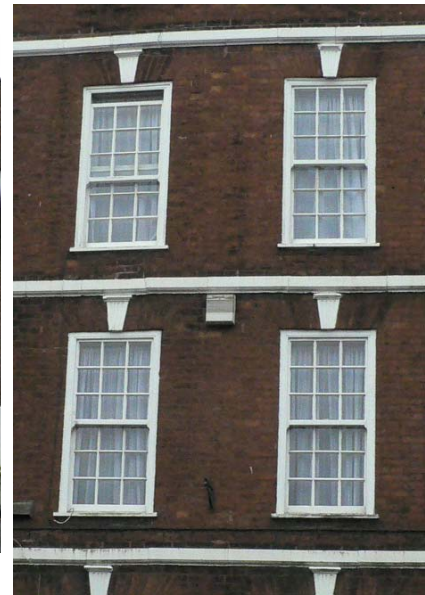
Nineteenth century Building with Six-over-six Sashes with Horns
