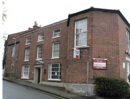
Brick Building with Sandstone Dressings and Plinth
