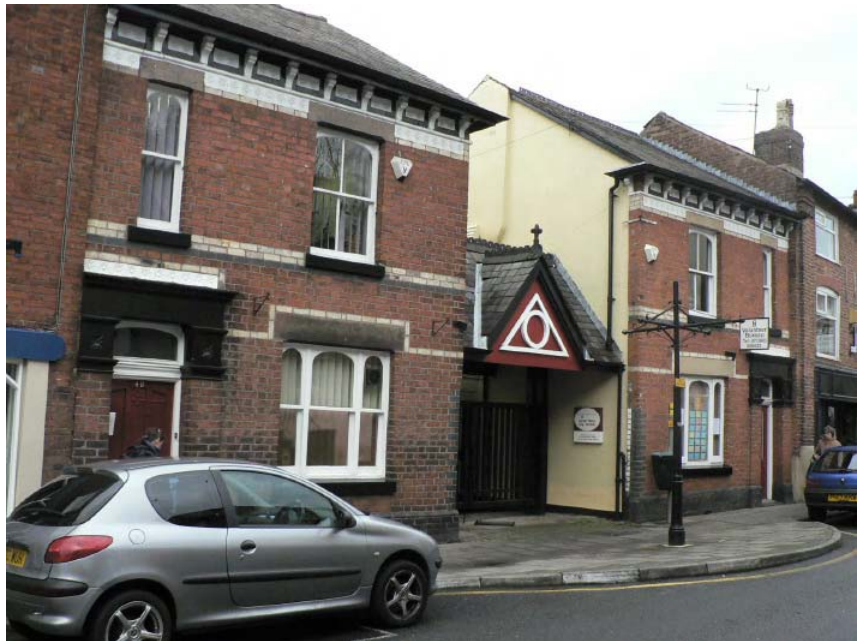
Intrusive Entrance to Carter House Day Services
