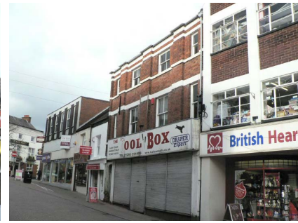
Early Twentieth Century Building
