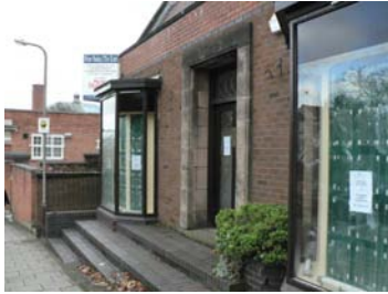
Vacant Building on Moody Street
