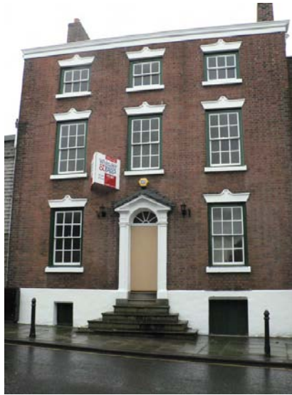
Georgian Building with Six-over-six Sashes without Horns
