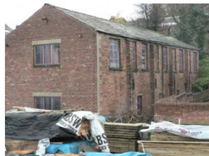
Nineteenth Century Building in Timber Yard
